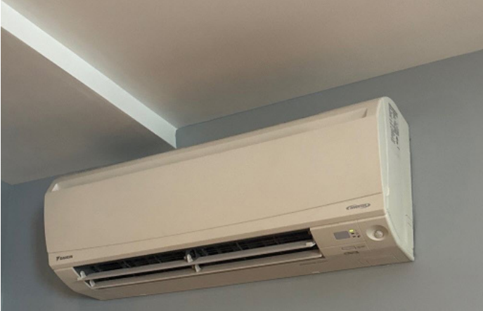
Unit Interior - Ductless Heatpump
